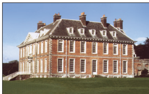
Uppark House - CF & CW System installed
